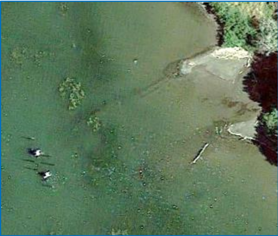
Figure 4. Pump Station Intake-Screen Structure into Pool (2022)
