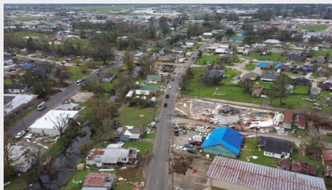
Hurricane Ida devastated Louisiana's bayou communities.
